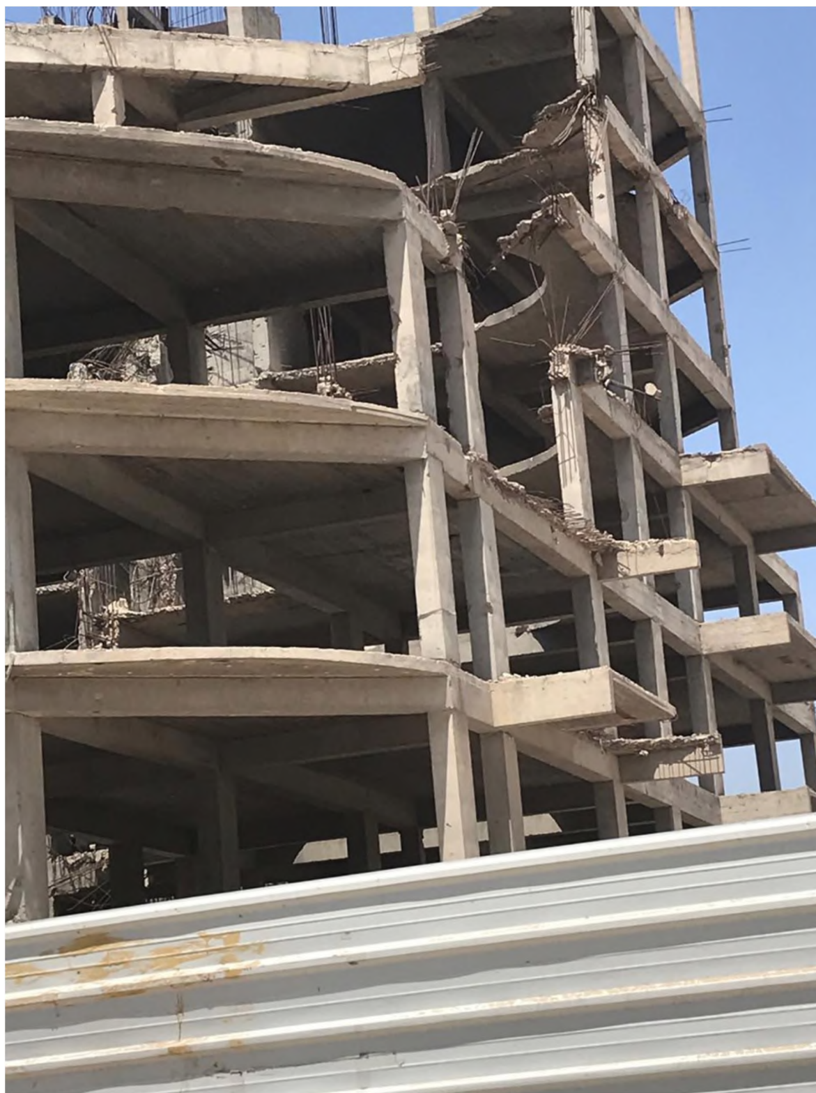
Fig. 2. The southeast facade of the commercial complex
