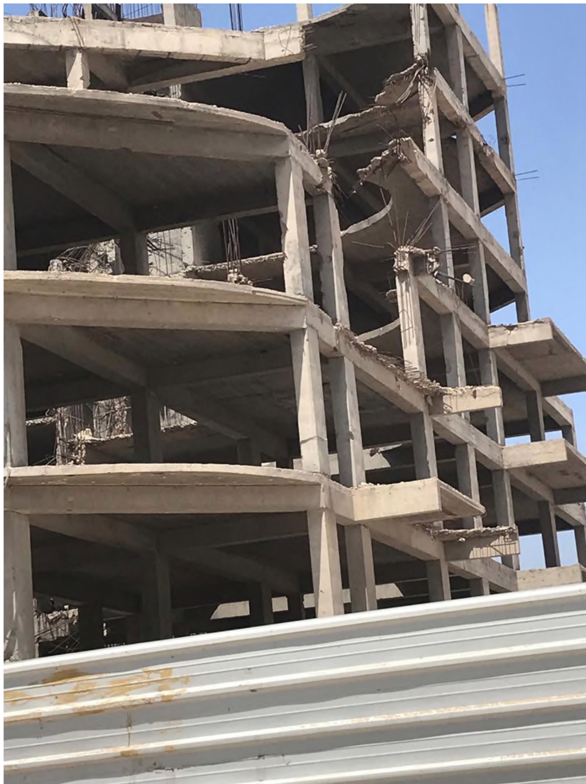
Fig. 2. The southeast facade of the commercial complex
