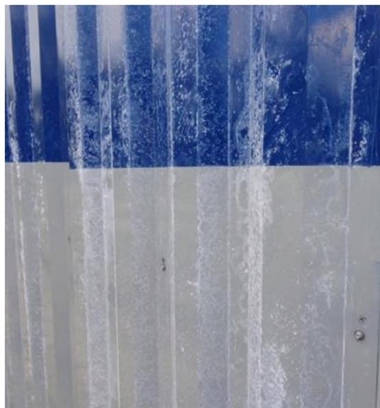
Figure 1. Violation of the integrity of the paint coating
