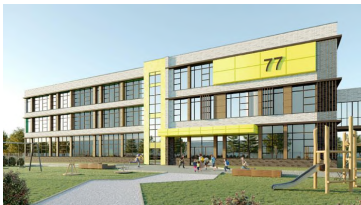
Figure 12. Main façade view
